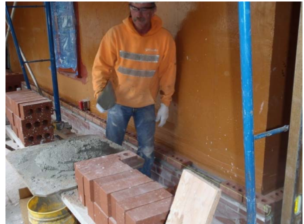
Brick: Stewart House Courtyard
