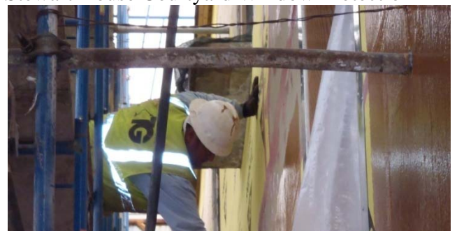
Stewart House: Waterproofing
