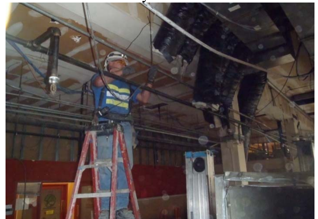
Electrical Work: Economy Market L7
