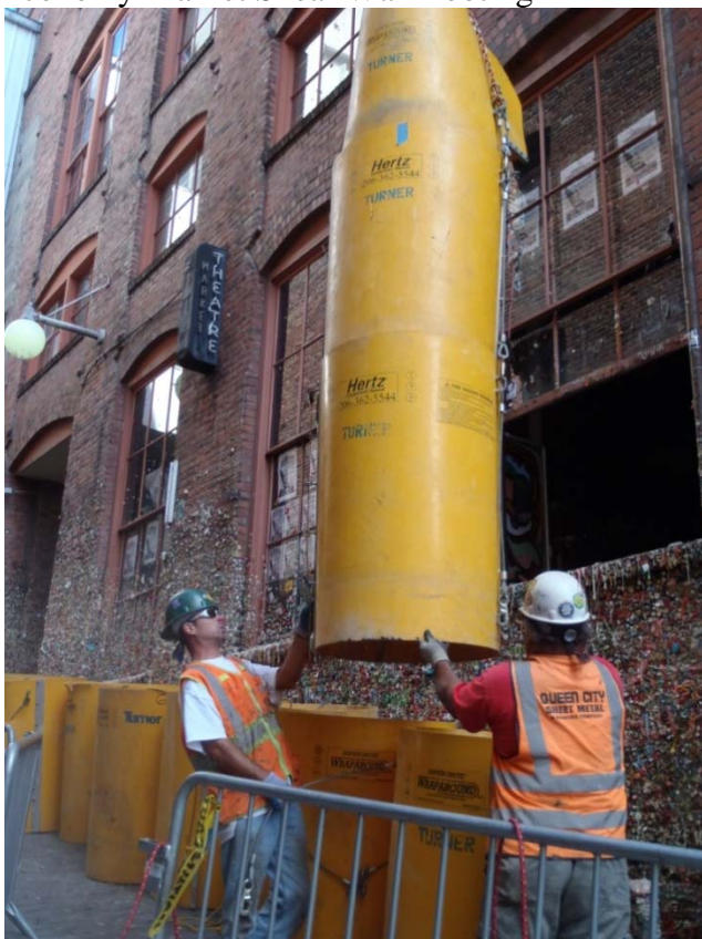
Building a trash chute Economy Market
