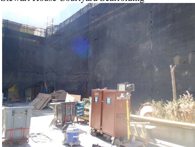
Scaffolding and Protective Netting in Stewart House Courtyard
