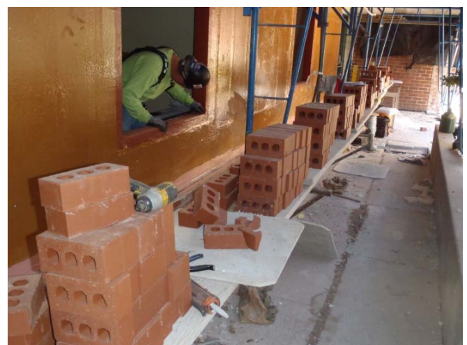
Laying Brick in Stewart House Courtyard
