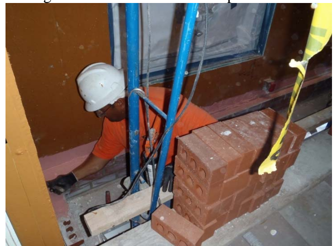
Cutting Brick for Stewart House Apartments
