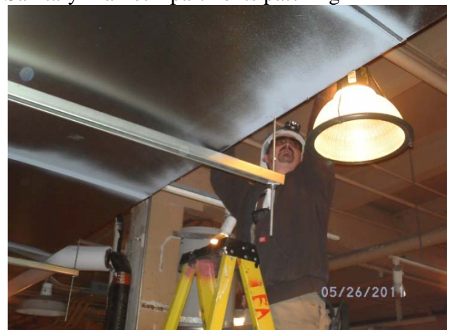
Shaft in Sanitary Market
