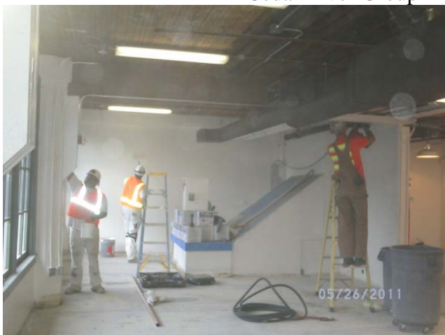
Piping and Painting in Cedar River
