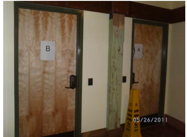
Bathroom Doors in Corner Market: Level 7
