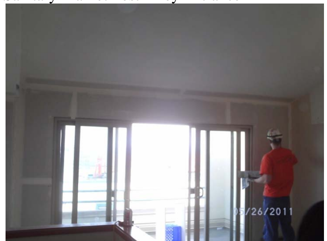
Sanitary Market Apartments patching
