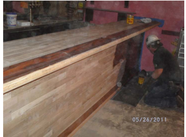
Finishing the new Can-Can Bar
