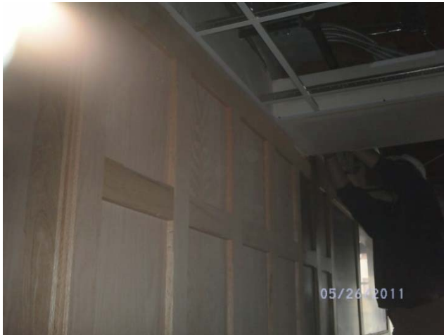
Wood Wall at Pike Place Bar & Grill
