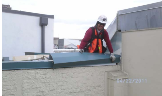
Corner Market Roof
