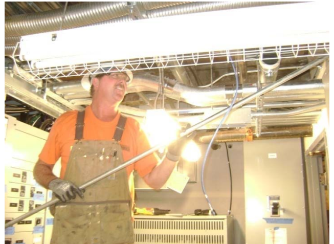
Laying electrical piping in the Sanitary Basement
