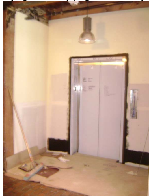
Elevator Lobby: Level 7
