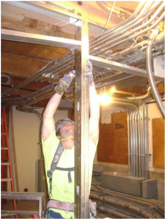
Framing Corner Market Electrical Room
