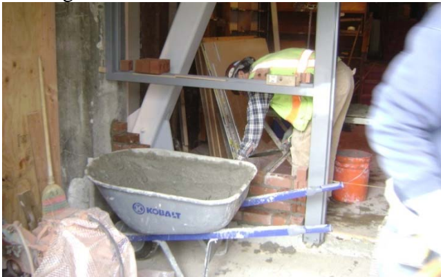
Installing brick around Left Bank Books
