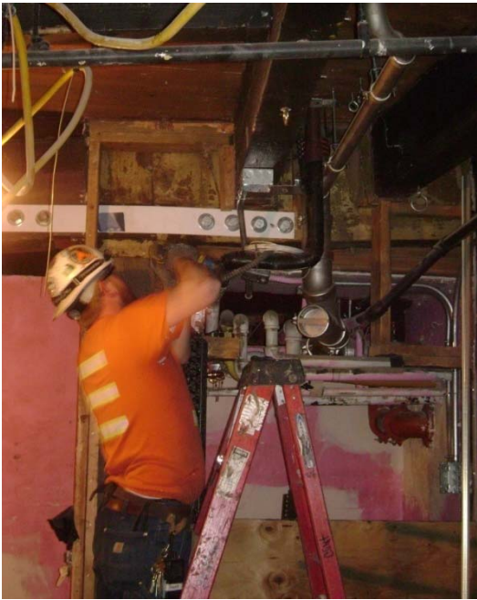
Electrical Work in the Can-Can
