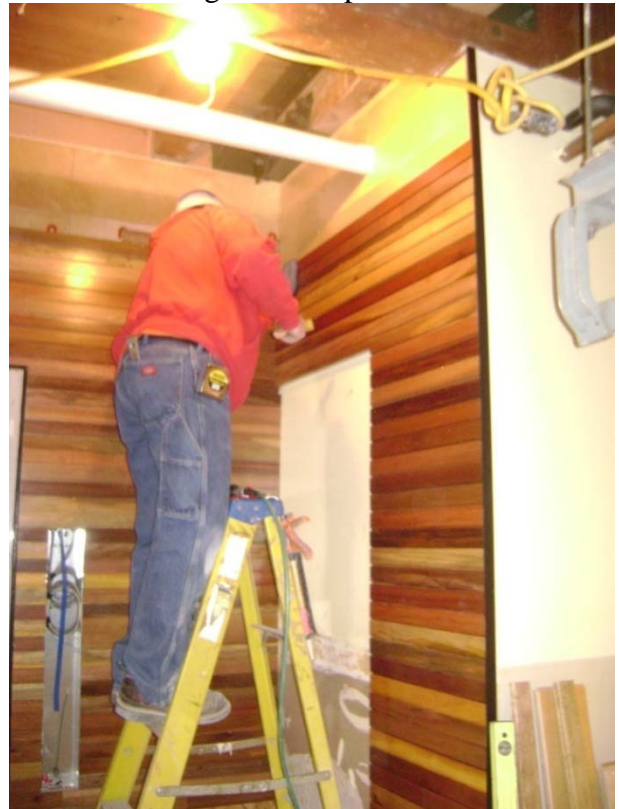
Installing wood paneling in Corner Market Elevator Lobby
