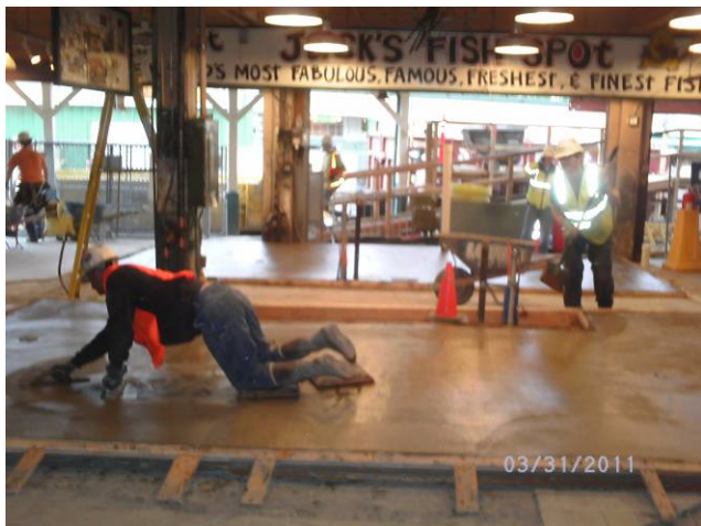
Jack's Fish: Finishing the new slab
