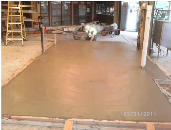
Jack's Fish: Finishing the new slab
