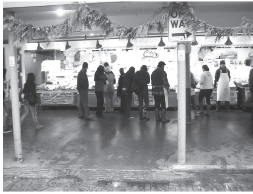
The new epoxy floor at City Fish. Pike Place Fish and City Fish will be closed for floor repairs in January.
