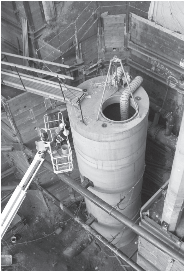
This new sewer manhole, located on the Market Hillclimb off Western Avenue, is 10 feet across and 43 feet tall. It houses sewer lines from the Market as well as the sewer main from First Ave. John Turnbull noticed that in this picture, the manhole resembles the world's largest soda can!
