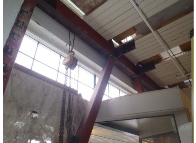
Brace Frame at Street level in Soames Dunn
