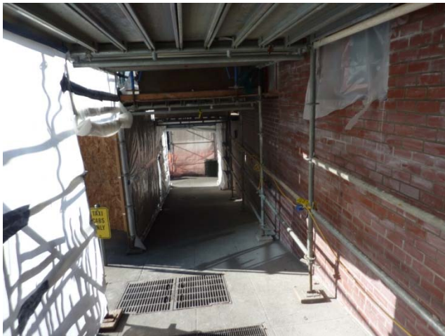
New brick on Stewart House
