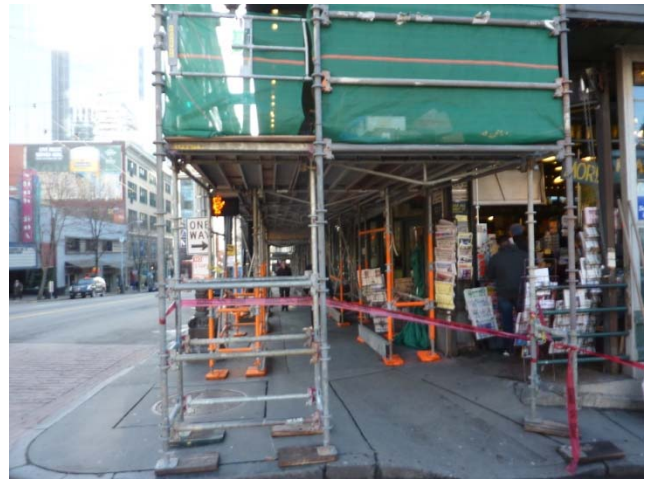
Scaffolding at Economy Market Canopy
