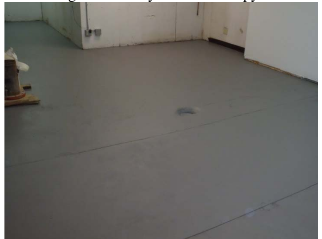
New Floor in Soames Dunn Basement
