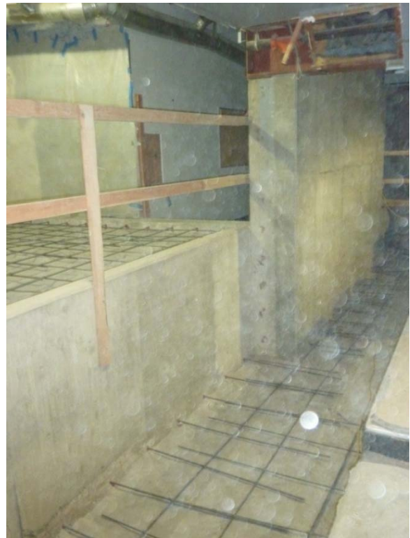
New Concrete work in Theater
