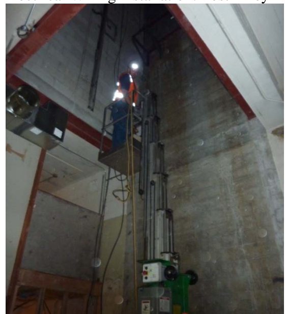
Soames Dunn Elevator Shaft
