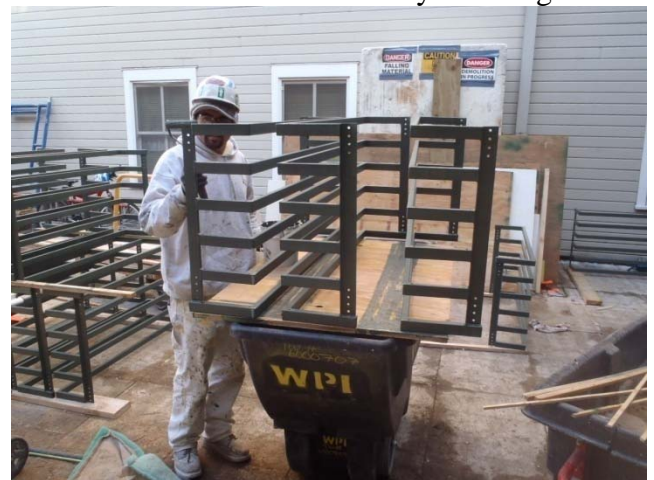
Balcony railing at Stewart House
