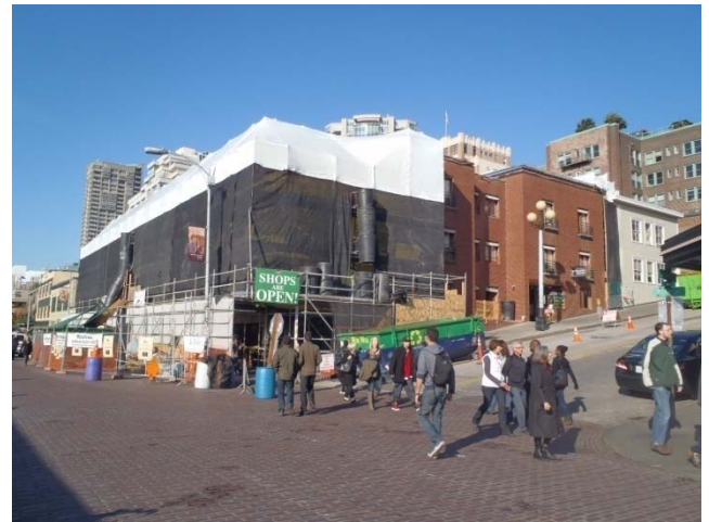
Stewart House Pike Scaffolding
